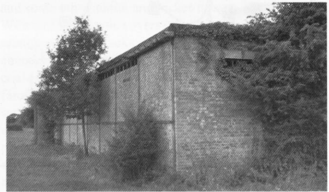
General shed construction view.
